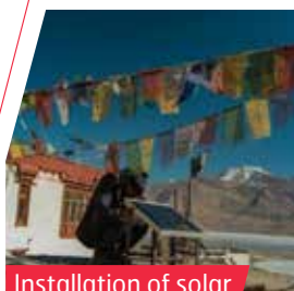
Installation of solar streetlights
